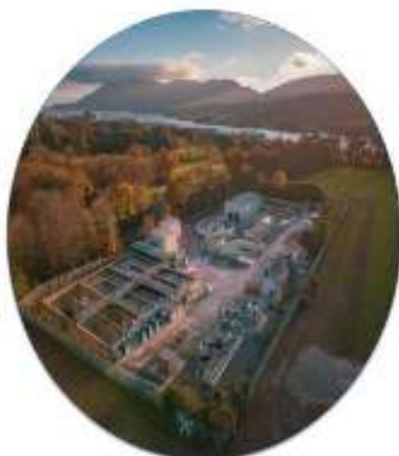
Warrenpoint WwTW £16m SWELL Project
