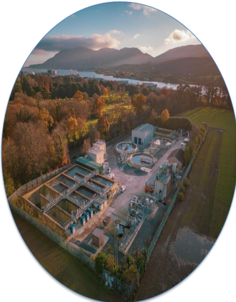
Warrenpoint WwTW £16m SWELL Project
