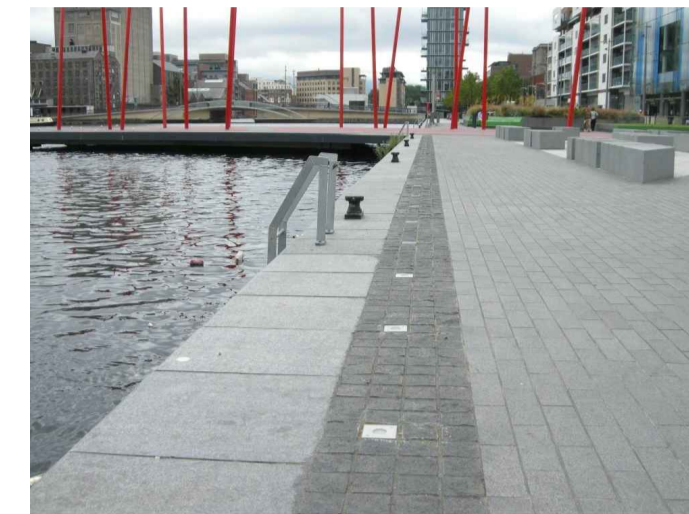
Illustrative image of re-formed formal interface with water, proposed as edge treatment to Plaza space
