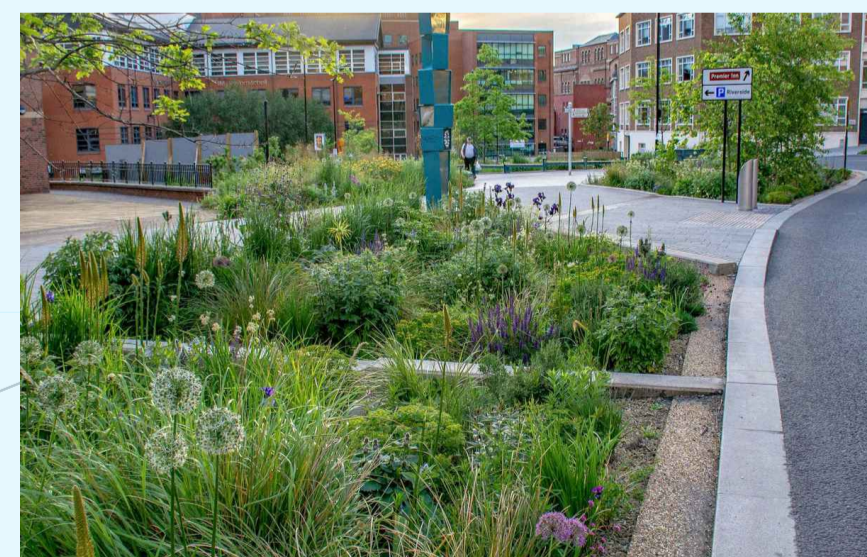
Illustrative image indicating potential for including varying drainage treatments (SUDs) within scheme
